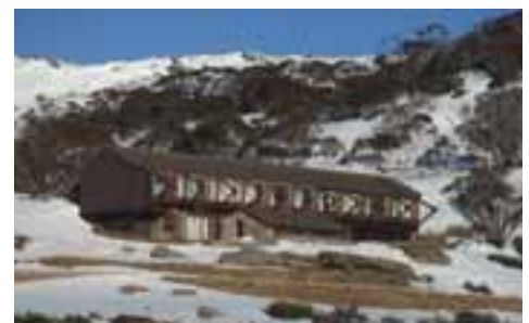
Yaraandoo during first stage construction (1962) and 50 years later.
