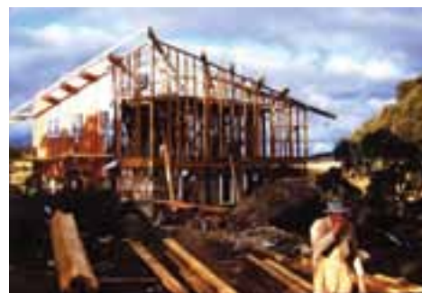
Ku-ring-gai Alpine lodge under construction in summer 1961/62. Photo: Jeff Jonas
